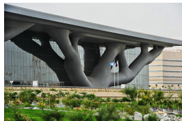
"Optimized" front-end of the Qatar National Convention Center.
