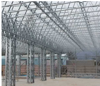
Example of a truss structure
