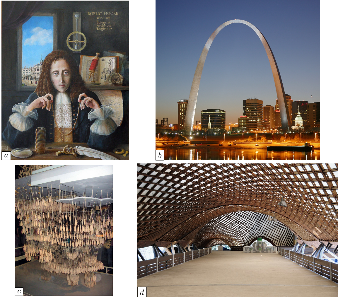
FIGURE 1.1.2. Shape optimization in architecture: (a) Robert Hooke with the catenary; (b) The St Louis vault (Missouri) is a “weighted catenary”; (c) Funicular model (assembly of catenaries) underlying the construction of the Sagrada Familia by Gaudi; (d) Optimization of the roof of the Olympic centre of Munchen (H. Berberich).
