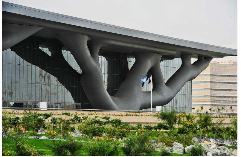
FIGURE 1. (Left) Shape and topology optimization of a landing gear by an industrial software (courtesy of Ansys ) (right) The Qatar National Convention Center (architect: Arata Isozaki) has the typical outline of a topology optimized structure (licence Creative Commons)
